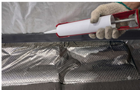
13/ Caulk the upper edge of the Wakastrap with an appropriate neutral-based roofing adhesive sealant.
