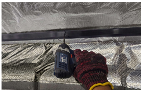
12/ Secure the Wakastrap to the wall.
