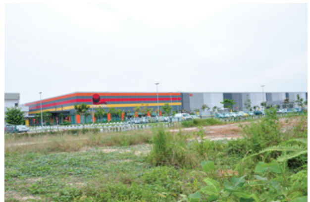
First Solar photovoltaic plant, Kulim, Malaysia
